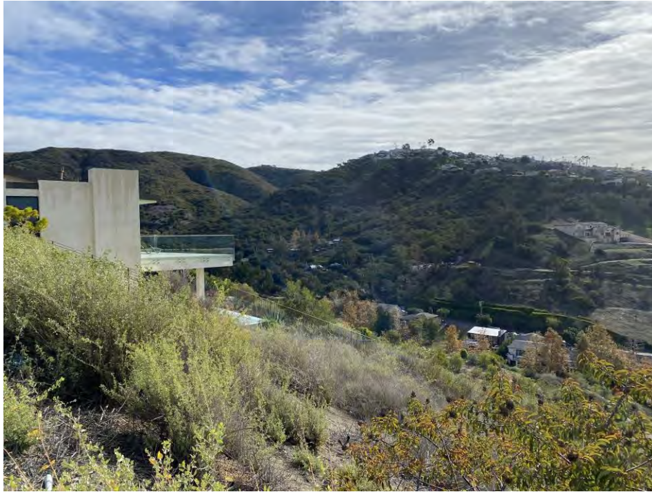
Photo 1: Overview east from Flamingo Drive toward upper Zone 18.
