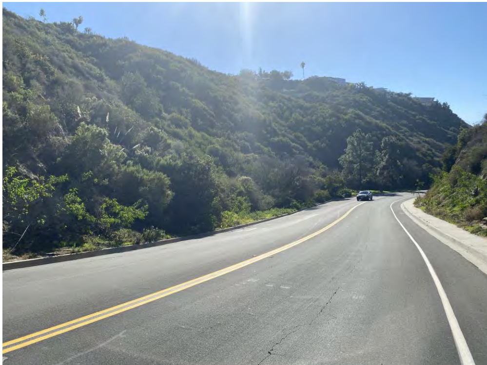
Photo 6, Middle Zone 22, view south
