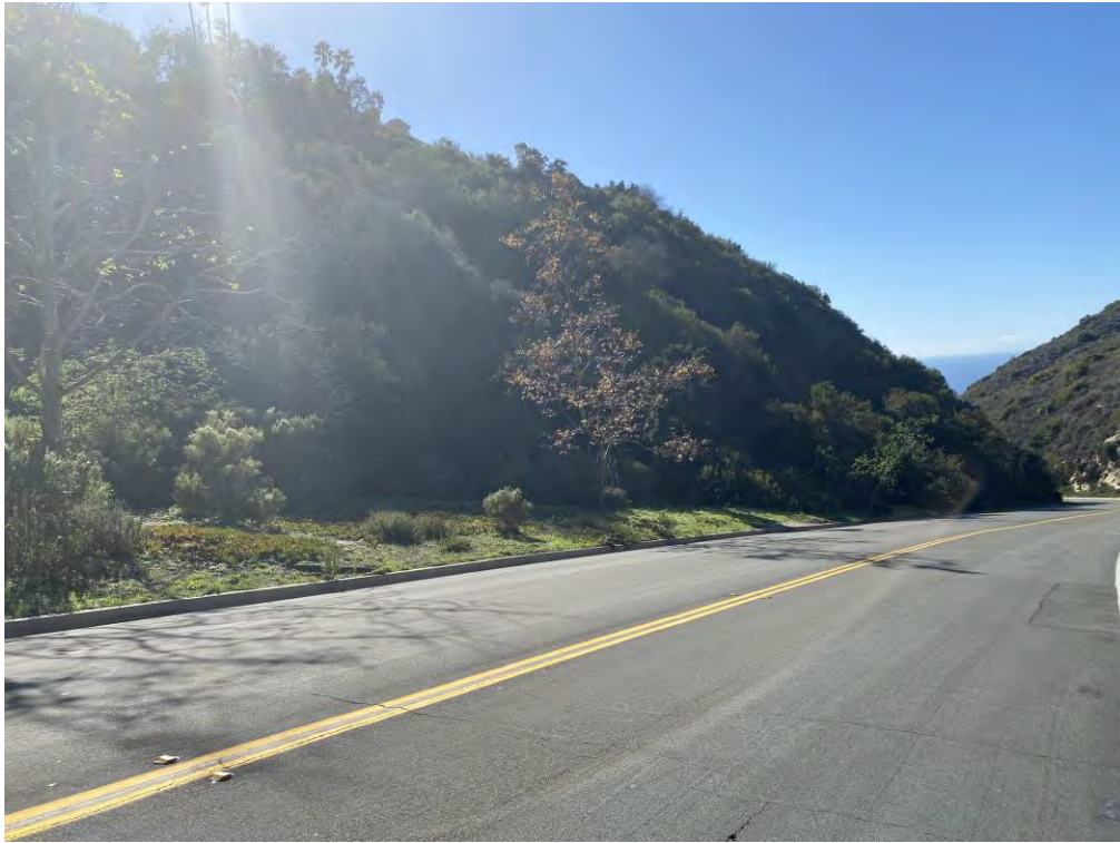
Photo 5, Middle Zone 22, view south
