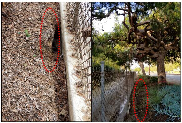
The top images are showing examples of where root expansion has begun to impact the channel wall; while the bottom image shows the collapsed wall and the large root mass located on the other side.
