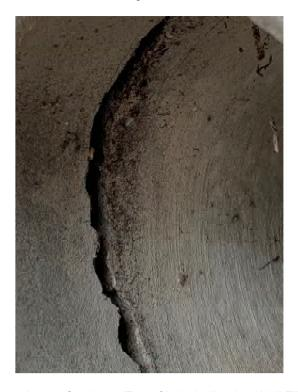
Photo 8 Large Cracks at Top of Inlet Indicating Wall Tilting
