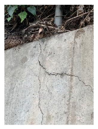
Photo 6 Cracks in Wall Adjacent to Tree Roots
