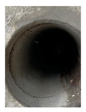
Photo 7 Cracking at Stormwater Inlet
