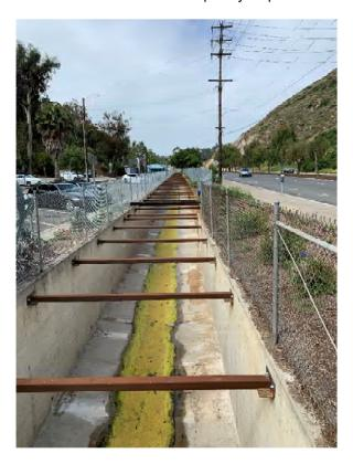
Photo 2 Shoring Installed to Reinforce Tilting Walls
