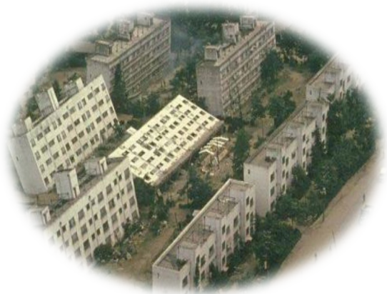
Liquefaction caused by the 1964 Niigita, Japan earthquake caused these apartment blocks to experience severe leaning. Image from the University of Washington.
