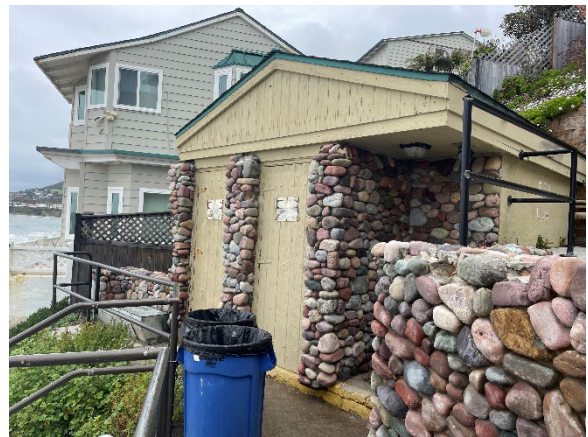
Photograph 6: View of pump station, looking north (Stantec, March 2023)
