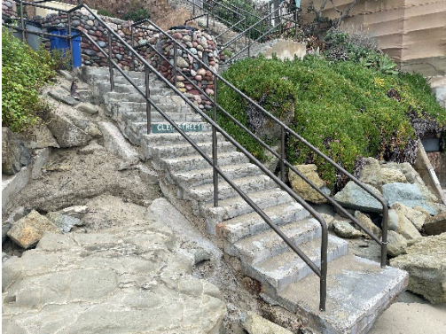
Photograph 1: View of Cleo Street beach access stair, looking south (Stantec, March 2023)
