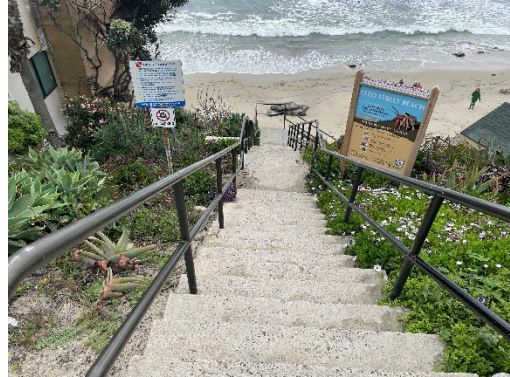
Photograph 2: View of Cleo Street beach access stair, looking west (Stantec, March 2023)
