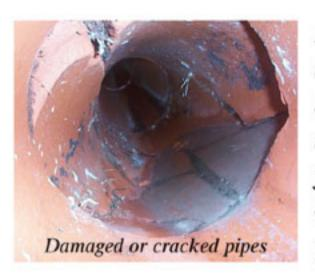
A private lateral that is structurally damaged and may also have separation of the pipe joints upstream or downstream of the problem.
